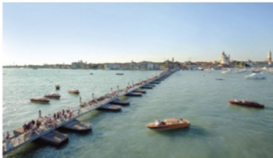
The temporary bridge for the Redentore Festival in Venice is a stunning example of the floating structures Ingemar helps develop for events.
