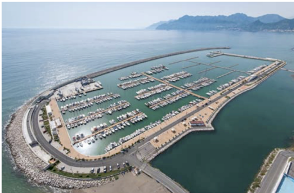
Marina d'Arechi on the Amalfi coast has boosted berths in southern Italy and is seen as a symbol of regional success.
