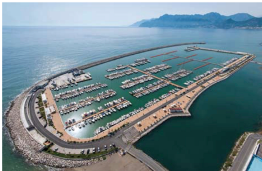
An Ingemar floating pontoon system at Marina d'Arechi in Salerno, Italy.
