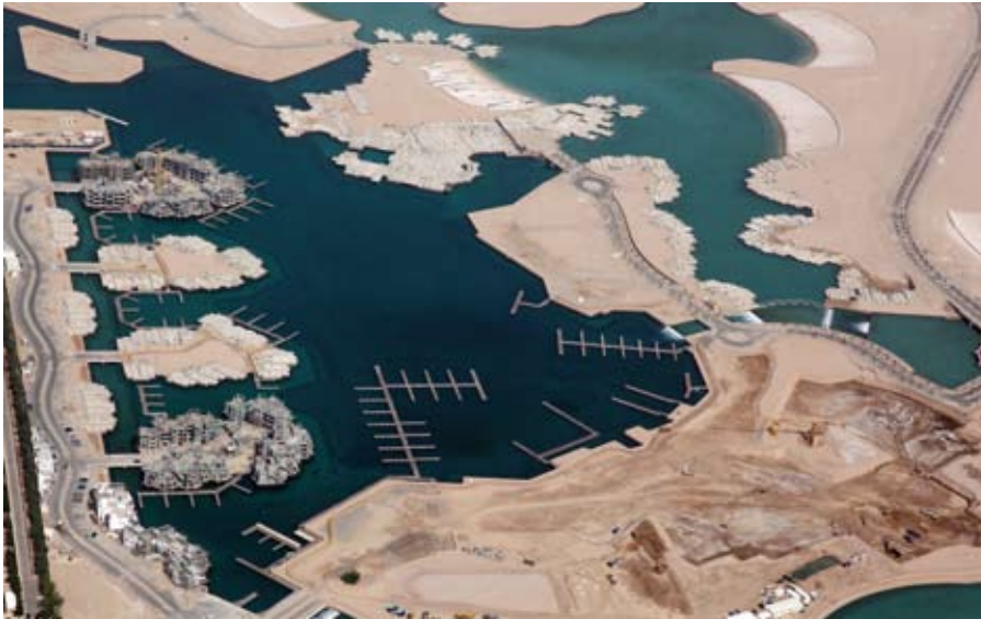
The pontoons and fingers for Ayla Marina in Aqaba, Jordan, have to fit an irregular quay profile.
