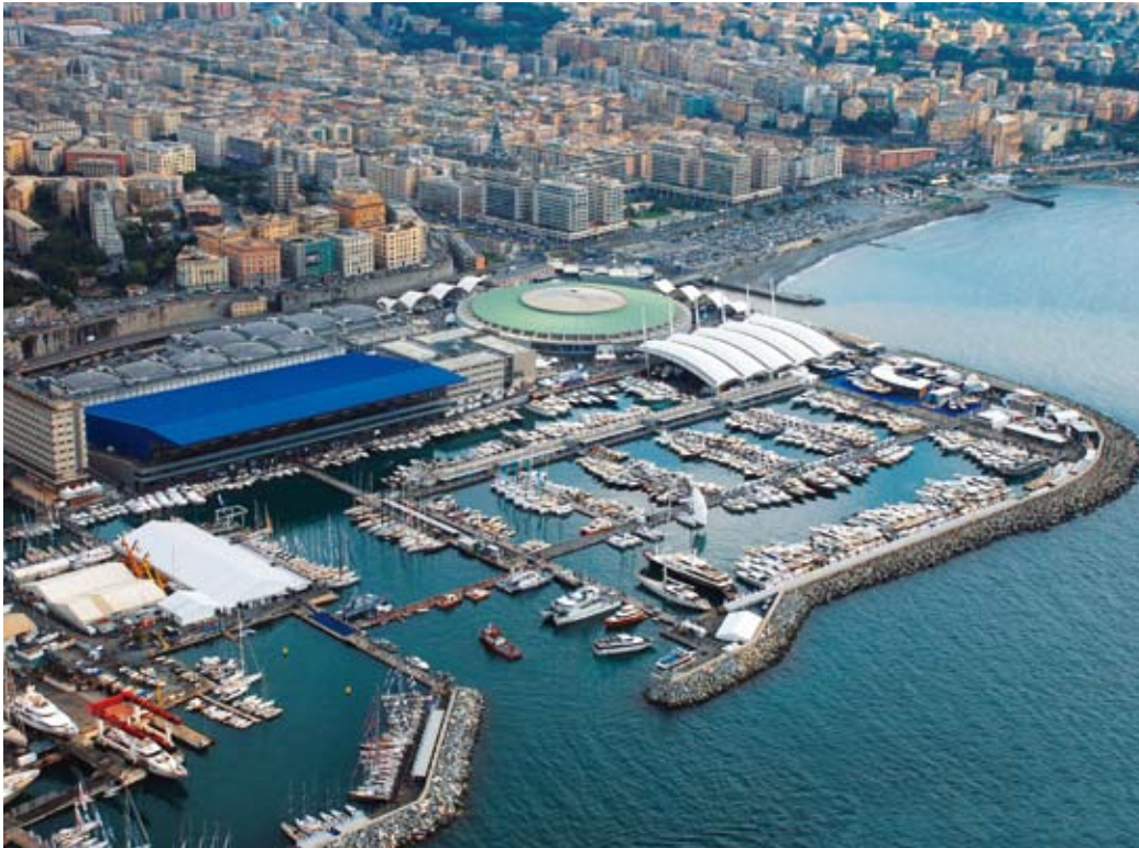
Ingemar supplies 10,000m 2 of floating jetties, platforms and walkways for the annual Genoa International Boat Show.
